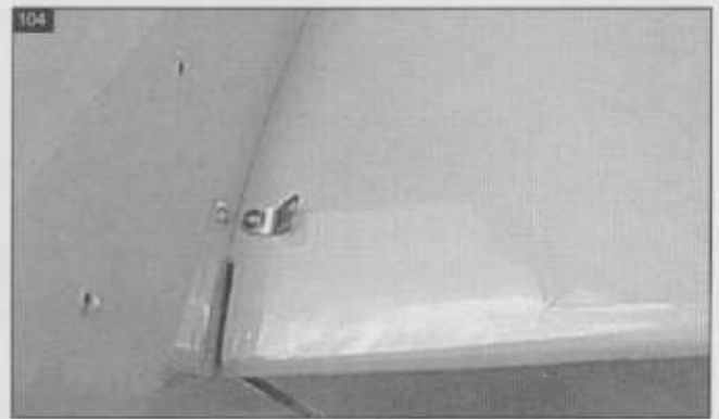
Install the metal strap.
